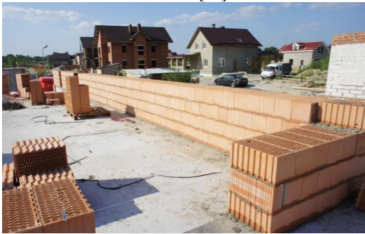
Figure 3 – Hollow ceramic blocks wall Source: [28]
