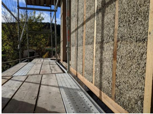
Figure 1 – Hempcrete wall performed by the tamping method Source: [26]
