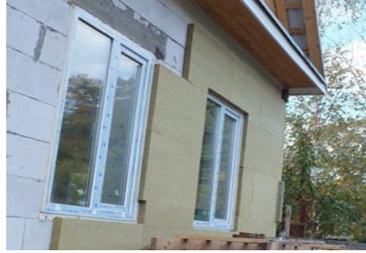
Figure 2 – AAC façade insulated with stone-wool wall insulator Source: [27]
